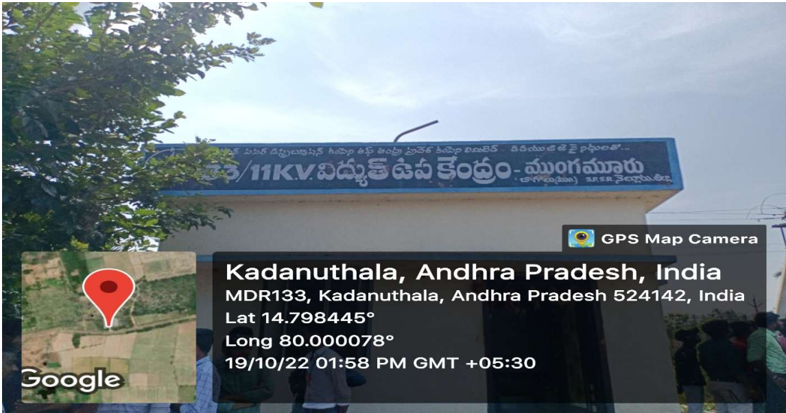
FIG: SUB-ENTRY FOR 33/11KV SUBSTATION, MUNGAMUR
