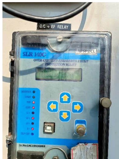
FIG: OVER CURRENT AND EARTH FAULT RELAY
