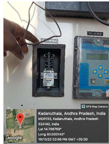
FIG: MASTER TRIP RELAY
