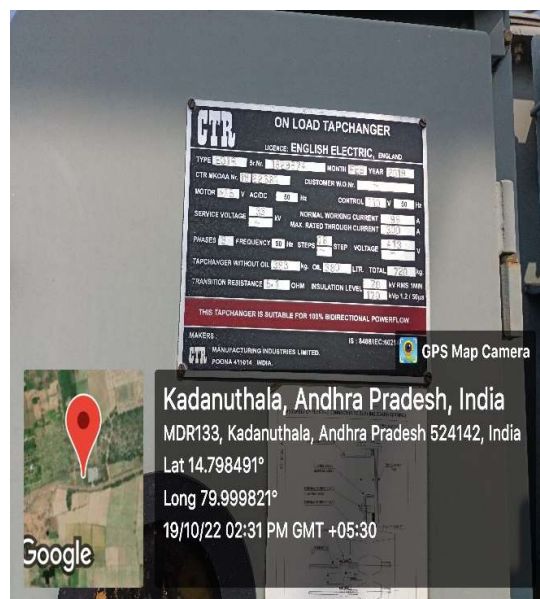
FIG: ON LOAD TAP CHANGER RATINGS
