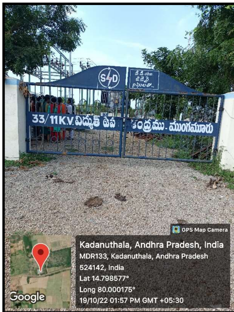
FIG: SUBSTATION MAIN ENTRANCE
