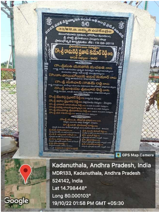
FIG: ENTRY NAME PLATE OF SUBSTATION
